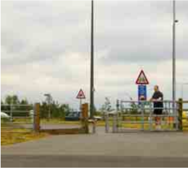
Example of barriers designed to prevent illegal use of a shared use route
