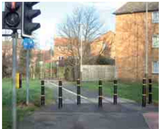
Example of route furniture designed to slow cyclists as they approach a road crossing
